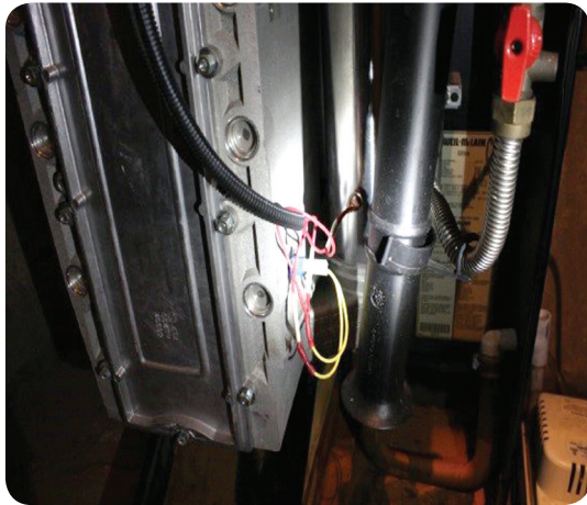
Figure 8 M6 sensor (Upper sensor)
