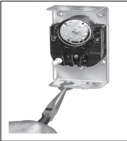
Fig. 5 - Removing slotted knockouts.
