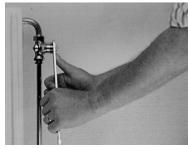
1. Using a 15/16" or 23 mm wrench, loosen the insert in the valve body by turning counterclockwise to break the metal to metal seal. Do not turn the insert out. Turn it back clockwise, tighten it lightly, if needed to prevent any objectionable leakage.
